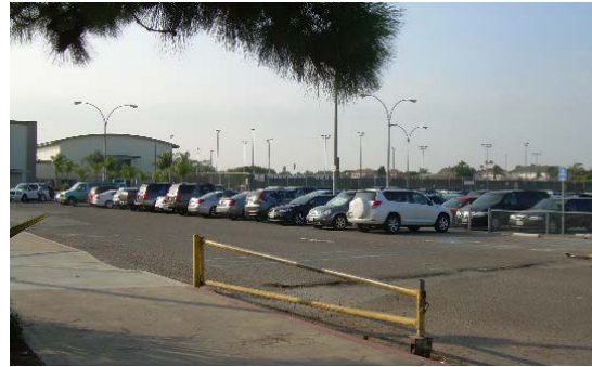
Major vehicular parking and circulation problems at student lot.
