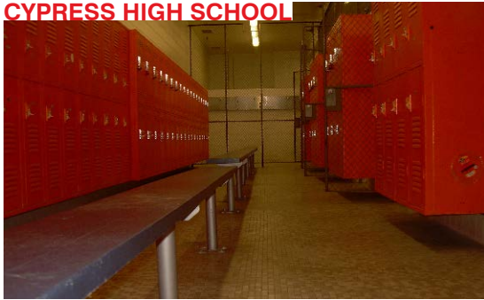
Revamp locker rooms.
