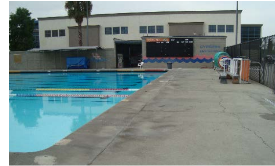
Pool in need of standard modernization.
